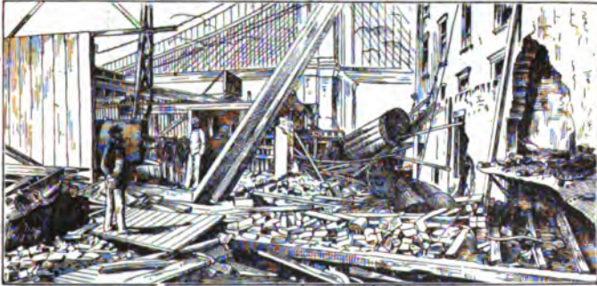
FIG. 158.—POSITION OF THE THREE BOILERS AFTER THE EXPLOSION.
